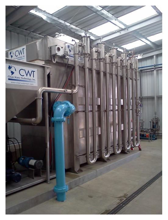
Figure 7. The GEM System installed at the rendering plant
